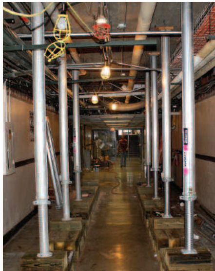
Steel beams support the sagging floors of the Natural History Building
